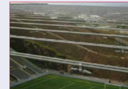
Braga Stadium (Portugal)
